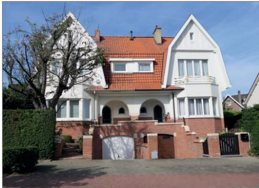
Figuur14: Grootveldlaan 246-248, arch. W. Minnigh, 1939 (ACWSP, ref. PU)
